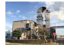
Hydrogen power plant
